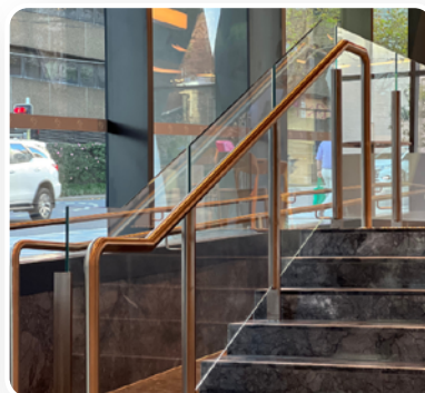
Stair Glass Balustrade – Stand-offs and Spigots
